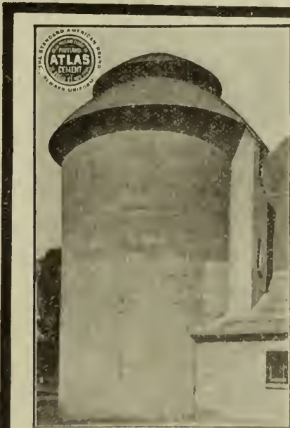
A CONCRETE SILO Gedney Farms, White Plains, N. Y.
